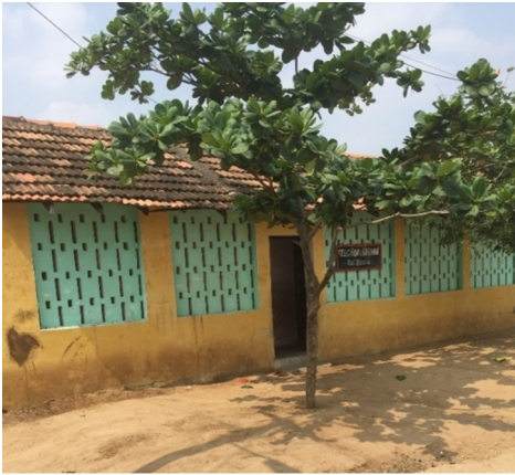
Figure 9 Renovated T.E.L.C. School
