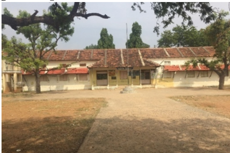
Figure 20 Board High School, Kamuthi—2017, same building even after 60 years
