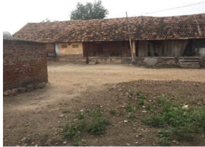
Figure 22 Abandoned Rajaji Hostel– 2017
